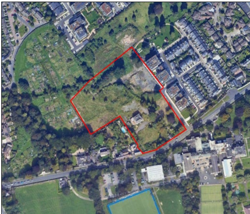
Figure 2.2: Indicative Site Location - Site outlined in red. (Source: Google Earth, annotated by Tom Phillips + Associates, 2024).
